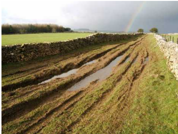
Photo: Damage to Minninglow Lane. January 2012
