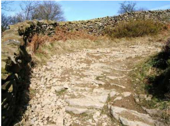
*Photo: WashgateLane. Damaged cobbles in March 2011. This picture was taken before the repairs were done by volunteers*
