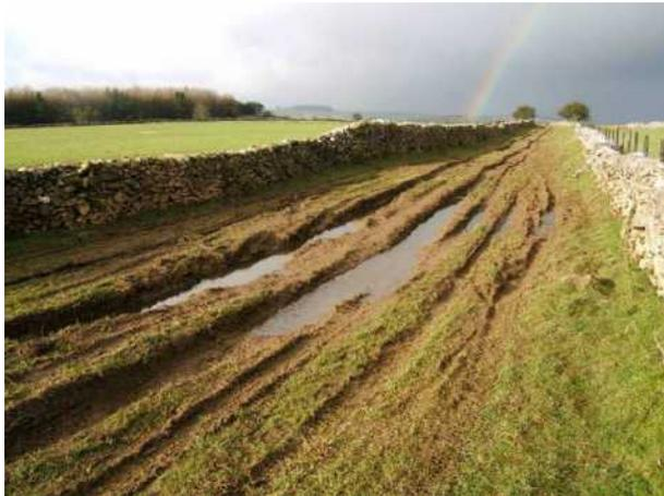
Photo: Damage to Minninglow Lane.
