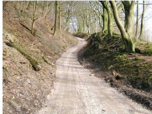
After DCC repairs March 2012
