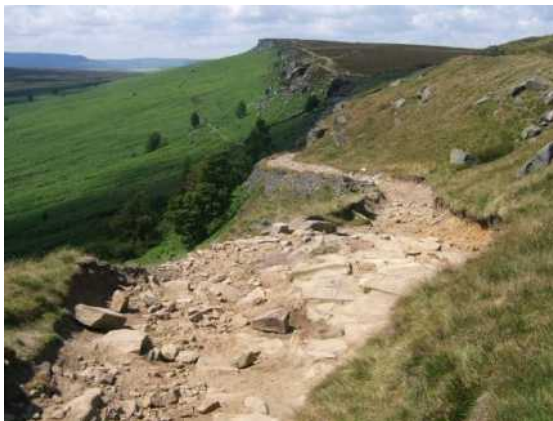
Long Causeway – Damage plus natural beauty. July 2011
