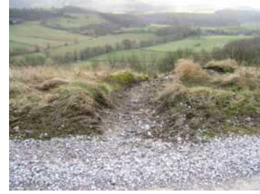
One of the many drainage channels created to solve the problem. January 2013
