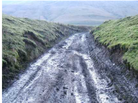
January 2013. The same area with the the grass dead and a mud rut eating into the bank.
