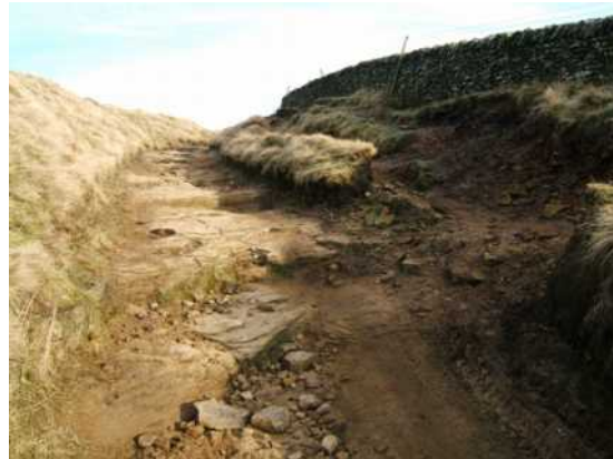
January 2013. A rock step when descending to the Sheffield Road. A parallel track has developed on the bank (not repaired by DCC)
