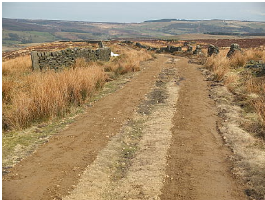
Part of the repaired section. Photo: March 2013
