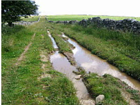
Water in ruts showing the drainage problems. July 2012
