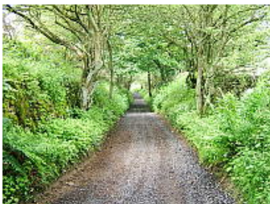
Bradley Lane after DCC repairs in June 2012
