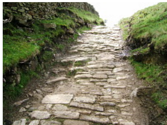
Pitching on the steep ascent to Roych Clough. Part of the £600,000 was spent on this work. Photo: June 2012
