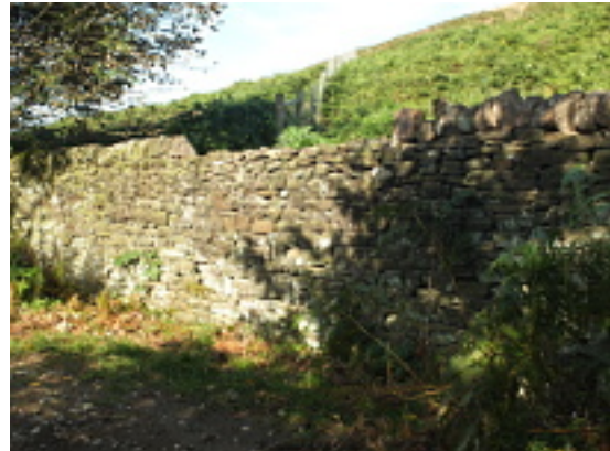
Loss of coping stones from the wall. We were told that off roaders have removed them to fill in ruts.
