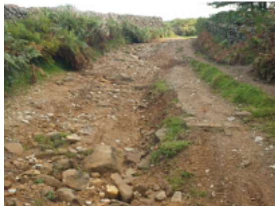
Water run off and tracks. September 2013
