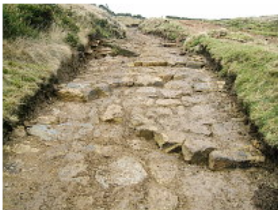
Repaired "bad step" area. December 2013
