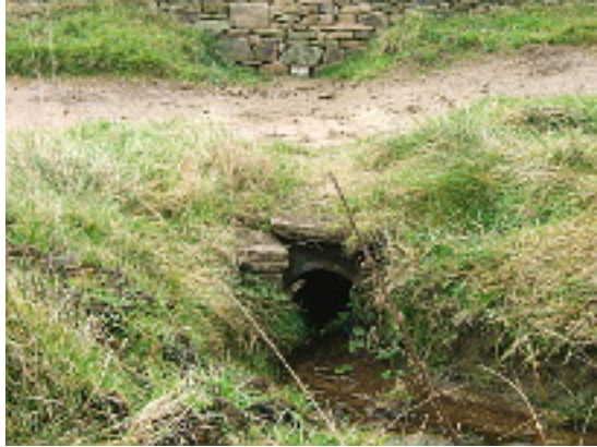
Example of new drainage. December 2013
