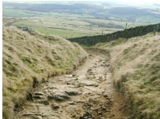
Unrepaired section between the junction with Beet Lane and South Head. December 2013
