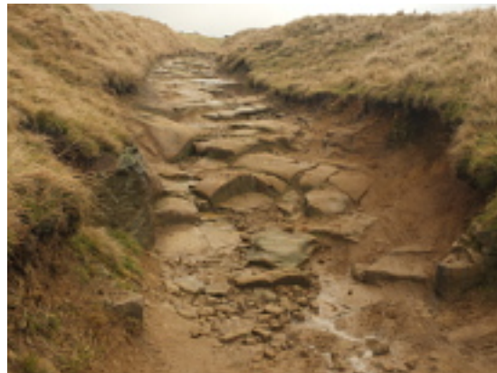
Many users find this section difficult. The TRO should help to reduce the rate of damage to this part of the route. Photo: January 2014
