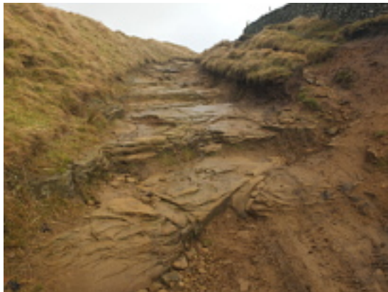
The steps in the bed rock on the descent to the Chapel Road seem to be increasing in height. Photo: January 2014
