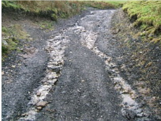
Water erosion is still a problem on the lowest part of the route in spite of the DCC repairs in 2011 and 2013. Photo: January 2014
