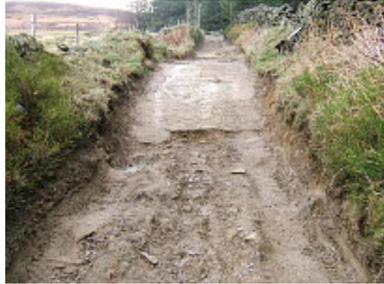
*Bamford Clough. Some of the concrete which is hazardous to all users when wet that DCC plan to remove. Photo: January 2012*
