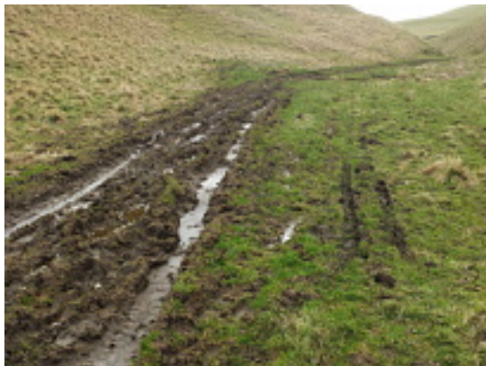
Widening of the track by vehicles. Photograph: February 2014
