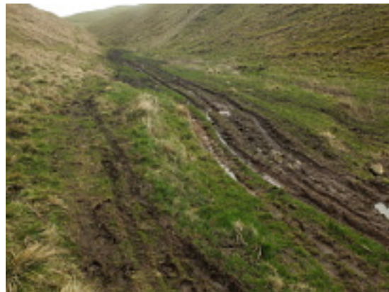
More widening of the track by vehicles on both sides of the route. Photograph: February 2014
