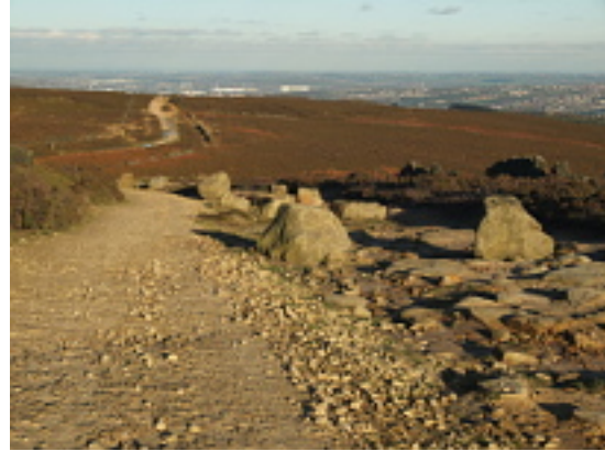
Houndkirk Road showing widening of the route in November 2013
