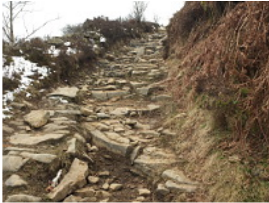
Leycotes Extension (Staffordshire part of Washgate) in February 2013
