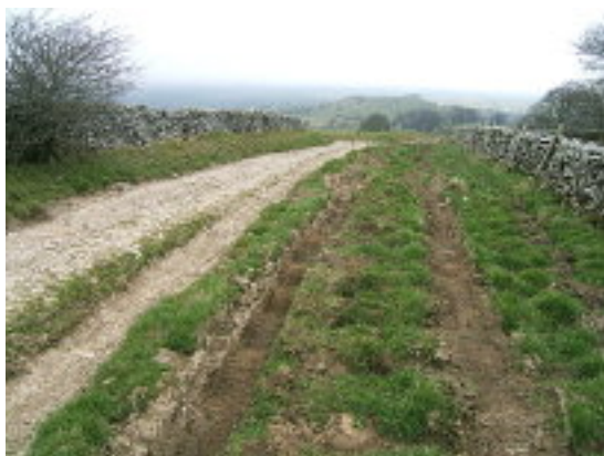
Some recreational motor vehicle users are using the verges even when the route condition is satisfactory.
