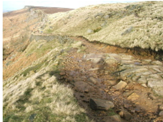
Damaged track and a view of the revetment in February 2014
