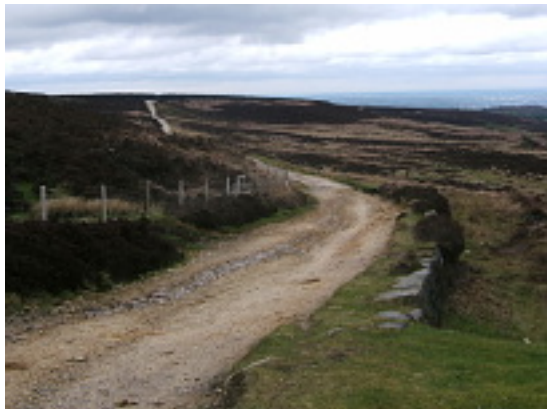
No signs of damage in May 2012 in the dip beside the raised track.
