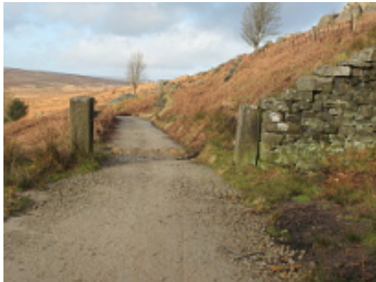
A repaired part of the route. Photo: February 2014
