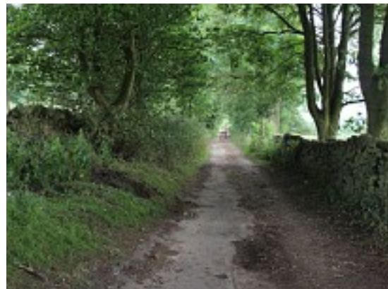
Photograph 7: The same area, repaired in July 2014
