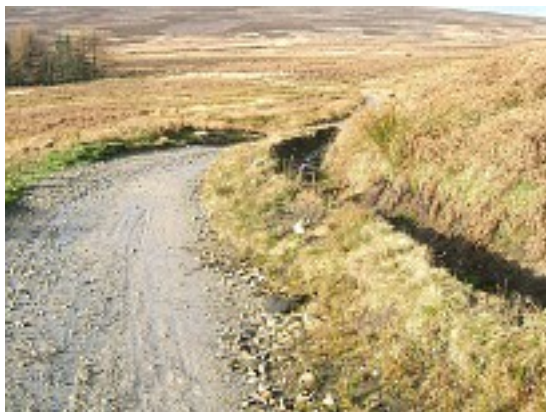
A culvert to take run off water. Photo: February 2014
