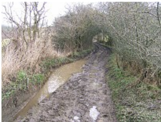
Just before DCC started the repairs in March 2012
