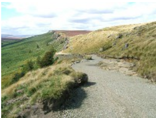
After the repairs in August 2014
