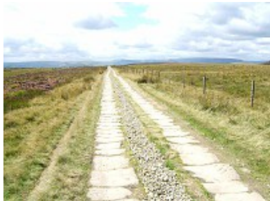
The repairs have sympathetically preserved the historic double causeway.
