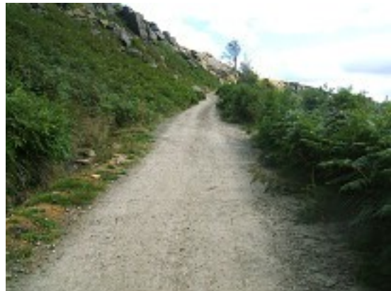
A similar area in August 2014 after repairs
