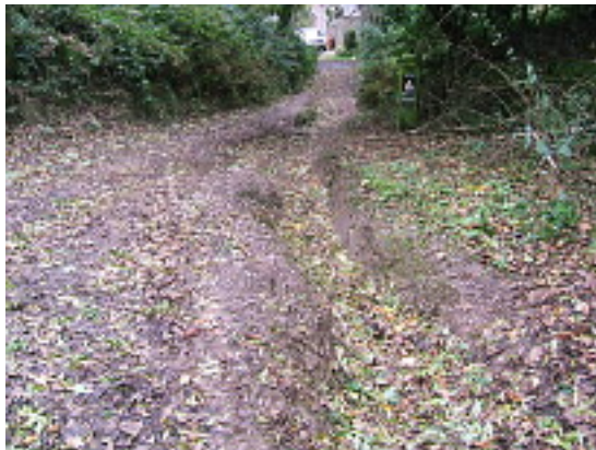
The deeply eroded section below the junction with Limer Rake looking towards Hollinsclough village. October 2014
