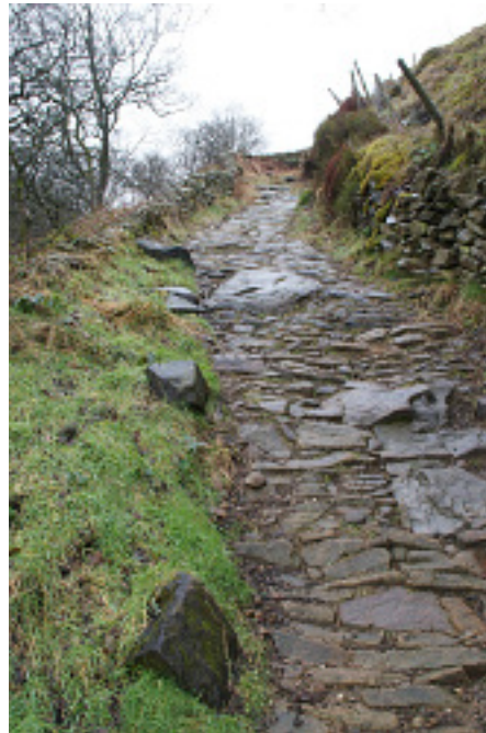
The Derbyshire descent to the River Dove, The setts have been repaired by the Peak Park Consultation volunteers: January 2015
