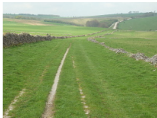
Taylor Lane. The white is where limestone chippings were placed in the ruts to repair damage caused by off roading. April 2014
