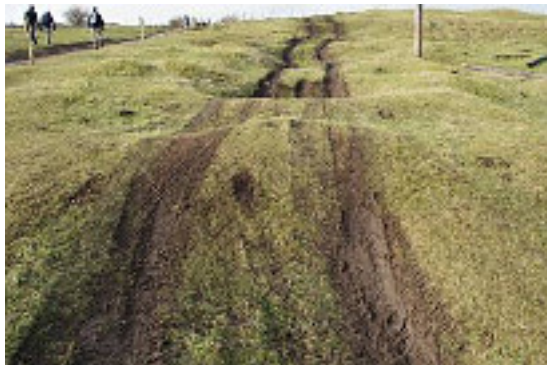
Damage to the historic lead mines earthworks on Putwell Hill. February 2015
