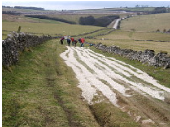
Working party in March 2011 showing the amount of limestone needed to fill the ruts.
