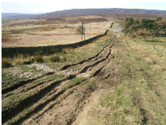
March 2014 - 11 months after the SCC repairs
