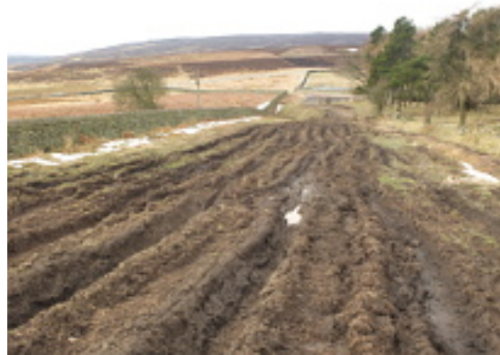
March 2013 before the SCC repairs
