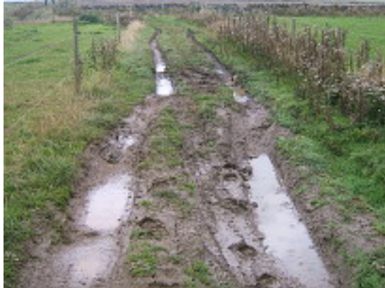
October 2015: Already showing visible signs of deterioration.
