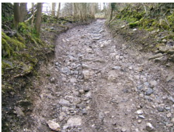
The condition of the steep uphill section continues to deteriorate. April 2016
