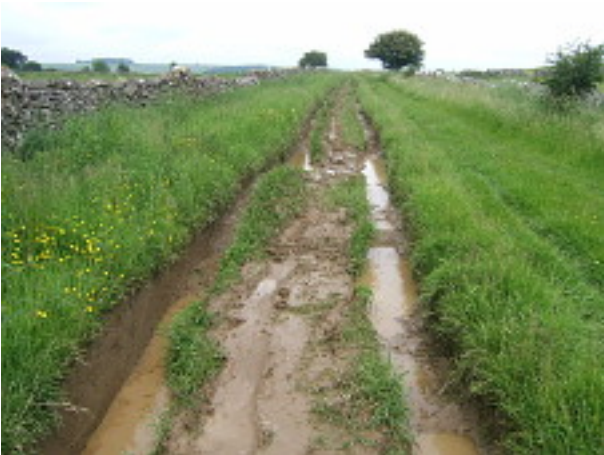
Photograph: Note the deep water filled ruts and the signs of vehicles “bottoming”. Some vehicles find driving along the ruts impossible and are using the remaining grassy section. Once ruts extend across the whole width, the route will become much more difficult for non vehicle users. June 2016
