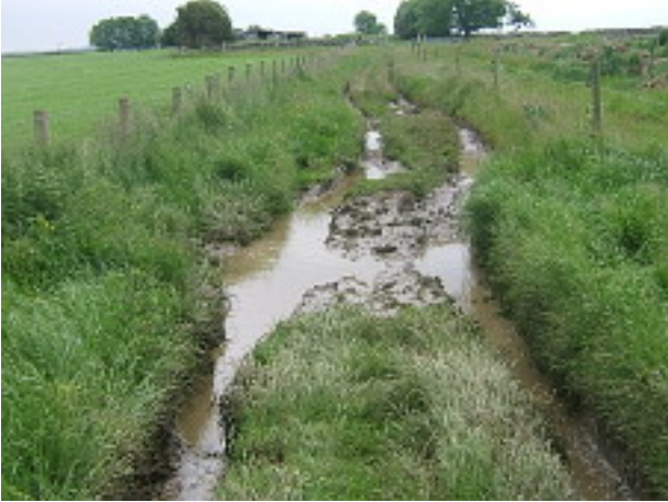
Route only passable by balancing on the narrow verges and avoiding the barbed wire and electric fence. June 2016
