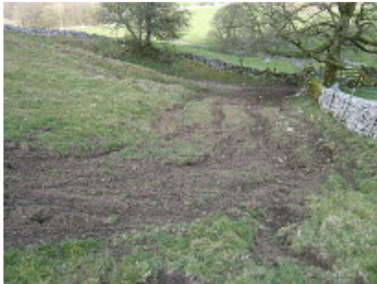
Off-roaders have created a scar on the hill side by cutting off a corner and driving over the humps and hollows of the hill. Sough Lane itself follows the wall which runs nearly horizontally across the photograph. April 2016
