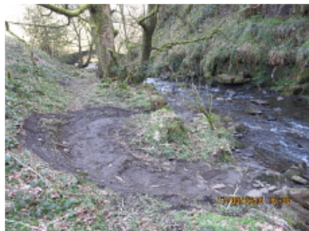
Damage on the Derbyshire bank. The photograph shows that motor cycles are riding illegally both on the bank and in the river. March 2016
