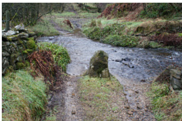
Photograph: The “ford” beside the packhorse bridge at the River Dove. The majority of motor cyclists cross the river here which leads to erosion of the river banks and the possibility of pollution of the river. January 2015
