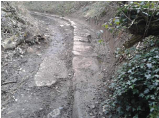
Remains of the causey. An alternative name for a causey, is causeway. It's made up of individual stone slabs laid in a line to provide a dry route over muddy ground; April 2016
