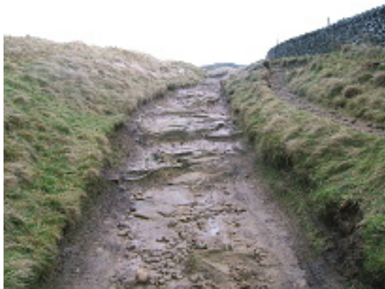
Steps with the alternative path on the right. Photograph January 2014.
