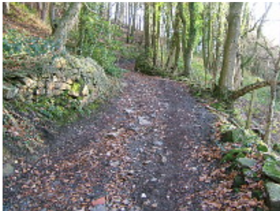
Damaged walls and bends: December 2015
