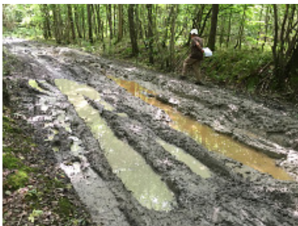
AE563 near Ruckinge. KCC plan to repair this BOAT. Photograph July 2016
