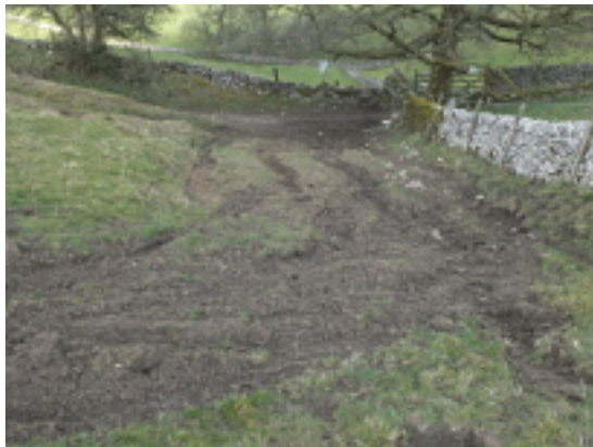
Near the gate at SK 131712. Damage from off-roaders cutting off a corner on a steep hillside. April 2016
