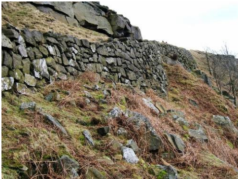
Long Causeway revetment from underneath
