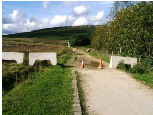
Barriers put up near Dennis Knoll to prevent 4x4s using the route during the closure
