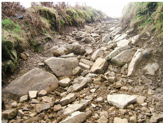
Loose rock and stone where Limer Rake has been eroded. February 2013
