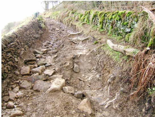
The fall beneath the exposed tree trunks was between 50 and 85 cm deep. February 2013
