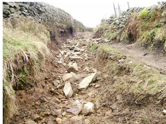
Near the bend at the top of the picture, the track is 90 cm below the wall footings. February 2013
