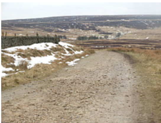
General view of Macclesfield Old Road: February 2013
