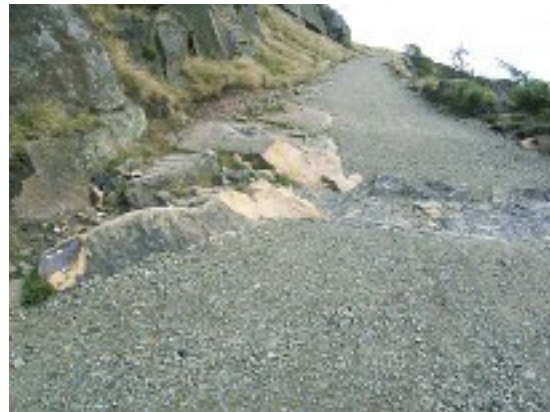
The same area in August 2014 after repairs
