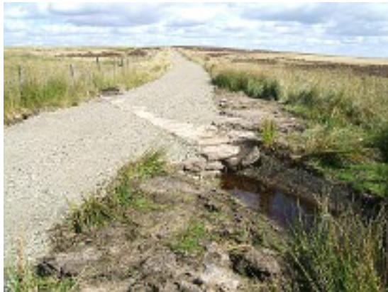
New drainage underneath the surface where a pipe leads water to a new "wetland area"
