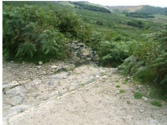
A new substantially built culvert across the path
