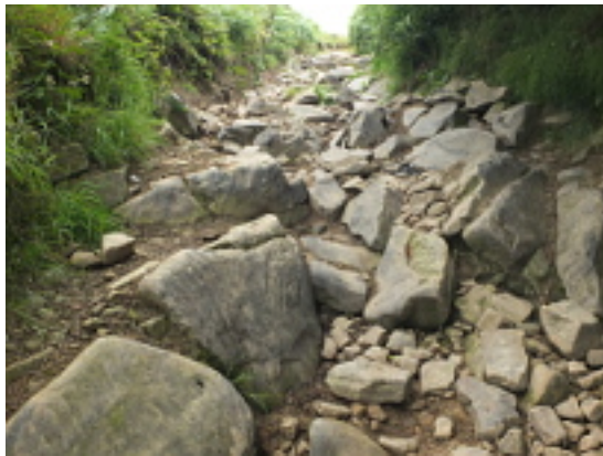
The steps on Limer Rake. Photograph July 2015
