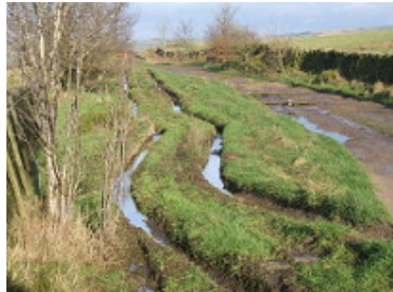
Extensive damage caused by vehicles driving on the verges of Over Hill Road. The nuisance is compounded by the fact that this section of the route is a restricted byway and should not be used by off-roaders. January 2016
