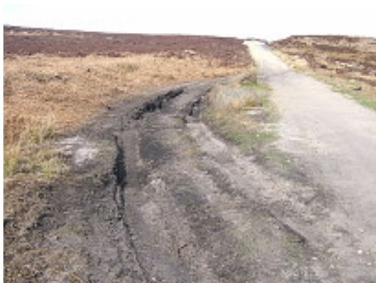
A "deviation" on Houndkirk Road. This "deviation" is not protected by boulders. PDGLA members have pictures of this off-piste activity from May 2014 and the ruts have been getting steadily deeper. March 2016
