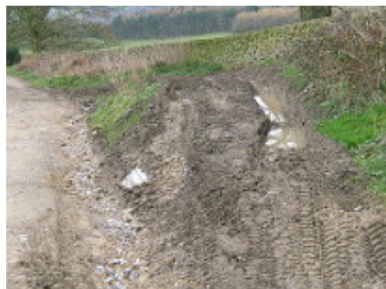
A small hillock on the side of the ORPA between Edensor and Handley Lane has been getting steadily more eroded with time. There are no problems with the surface necessitating this detour. April 2016
