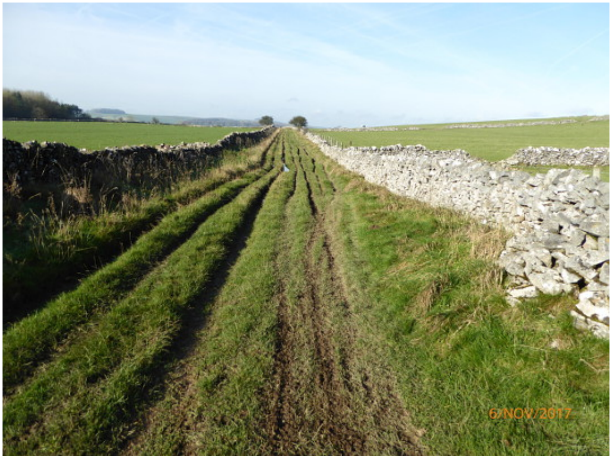
Part of the route on 6 November 2017. The narrow strips of ground between the ruts are very muddy, so walkers face slipping into the ruts. The strip next to the wall actually slopes steeply and in places has been churned up by vehicles. So although it looks green and pleasant, it is not easy walking.
