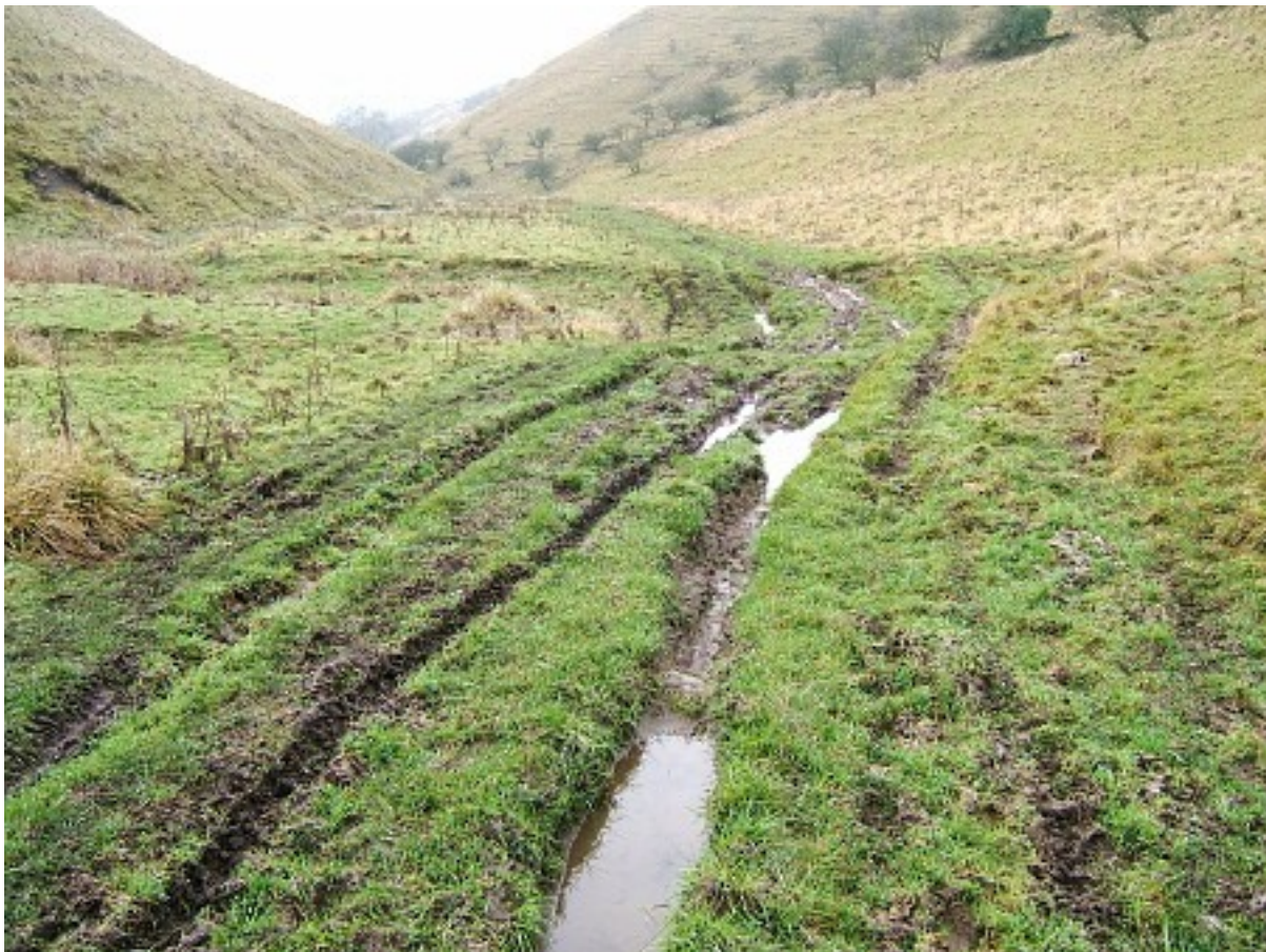
The middle section, heavily rutted, in January 2013
