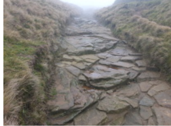
The stone steps have been retained. January 2020
