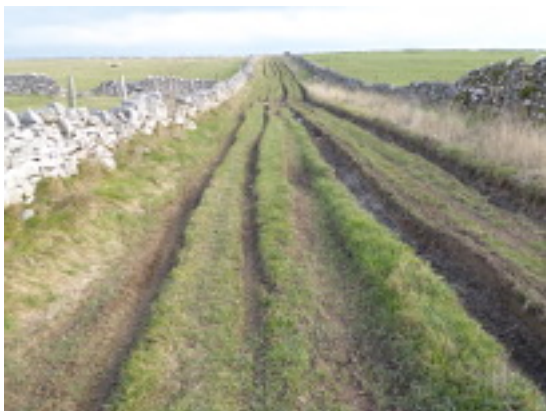
Before the repairs in February 2019
