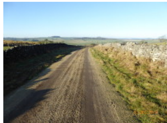
After the repairs in December 2019
